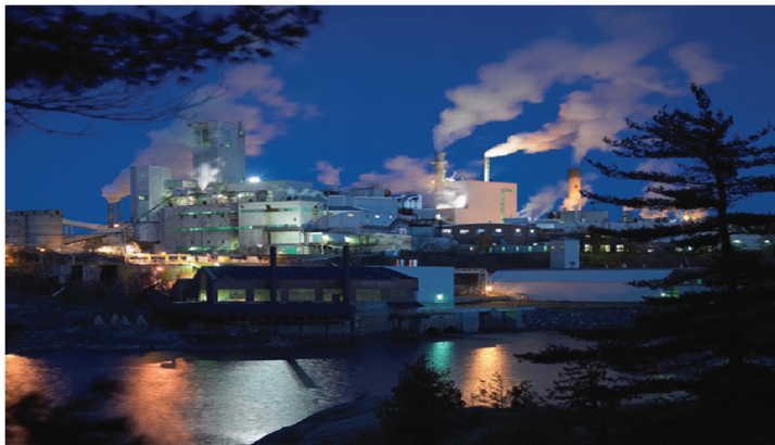
Figure 1: Domtar Espanola Mill
